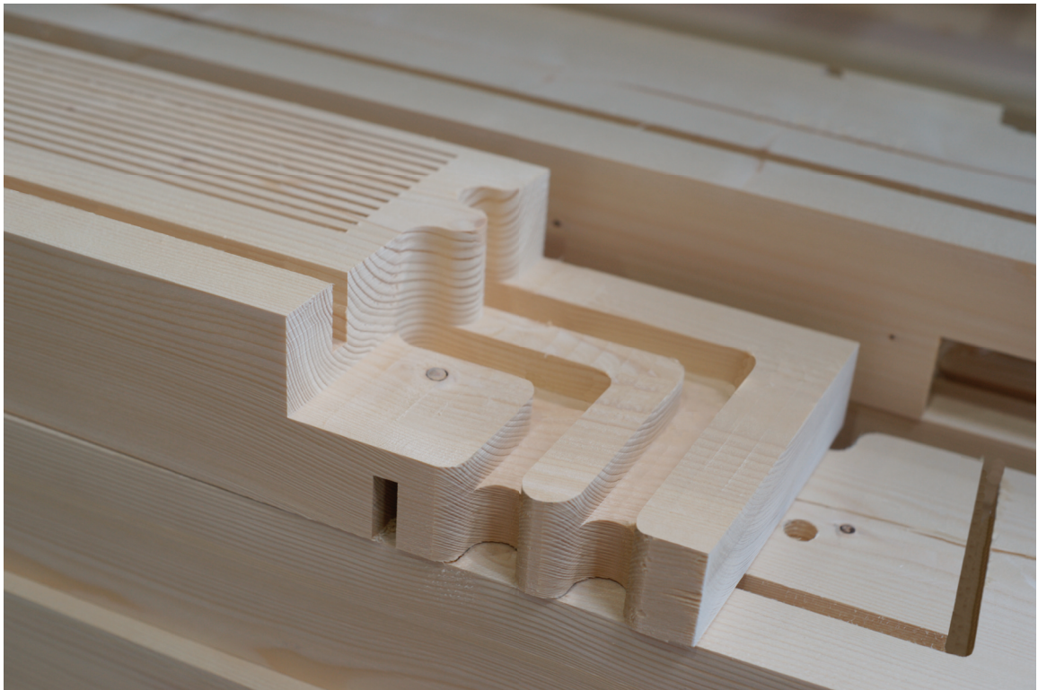
Timber Prototype House, Detail Eckverbindung / © ICD Stuttgart, Foto: Oliver Bucklin
