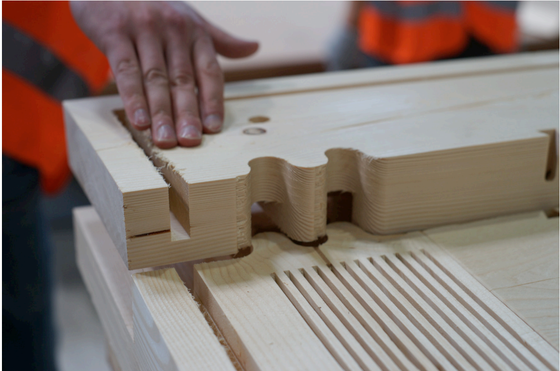
Timber Prototype House, Montage Eckverbindung / © ICD Stuttgart, Foto: Oliver Bucklin
